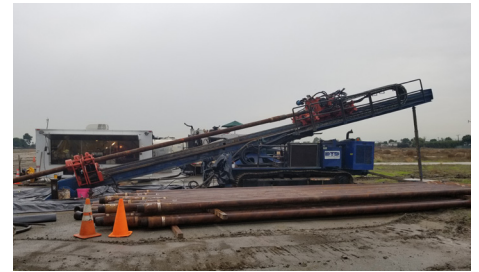
Horizontal Remediation Wells Drilling
