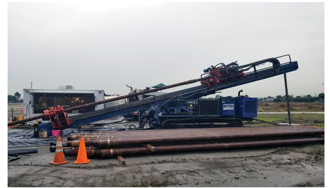
Horizontal Remediation Wells Drilling
