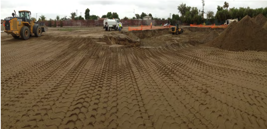
Photo 1: Backfilling, southern end of Excavation 3-4-14, view to the north.
