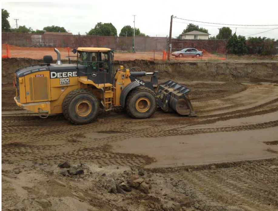
Photo 2: Backfilling, northern end of Excavation 3-4-14, view to the north.
