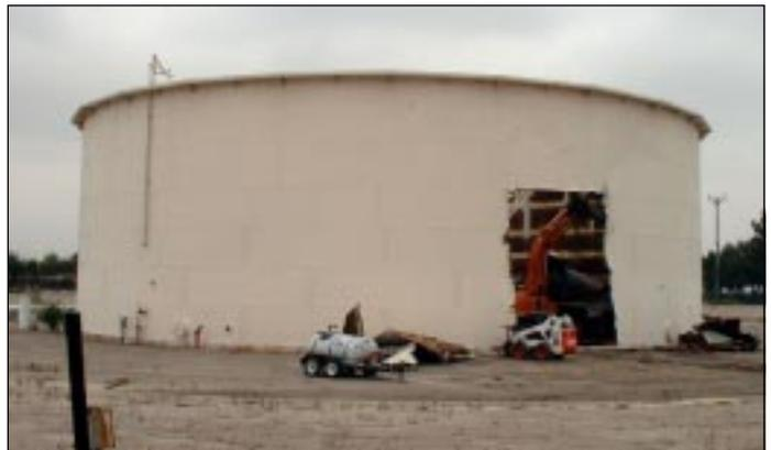
Completed Access Hole. The access holes cut into the tanks are large enough to drive a drill rig through to conduct soil sampling.
