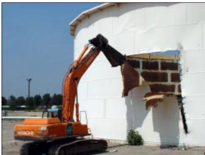
Cutting Open Tanks. A large shear cuts into the first of three tanks.
