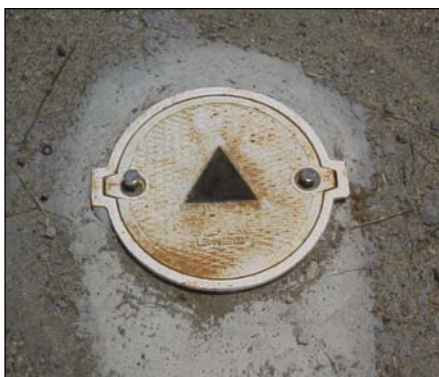
Other monitoring wells at the Tank Farm have caps at ground level such as this one.
