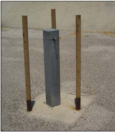
Some monitoring wells located inside the Tank Farm have aboveground caps.
