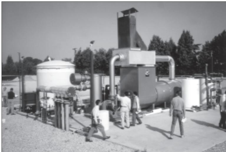
DESC's cleanup system in the central area of the Tank Farm is shown here during a recent site tour. It has a recovery rate of 1,000 gallons per month.
