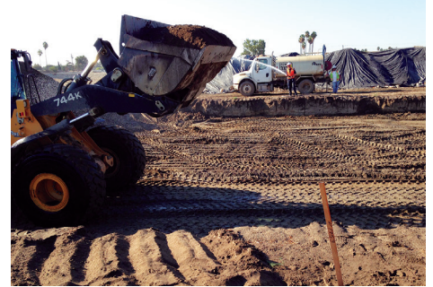
Backfilling of Excavated Area
