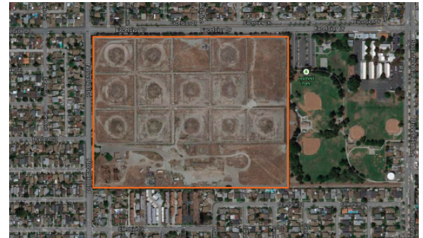
Current Aerial View of Former DFSP Norwalk Tank Farm Site, Post-Removal of All Tanks and Fueling Stations
