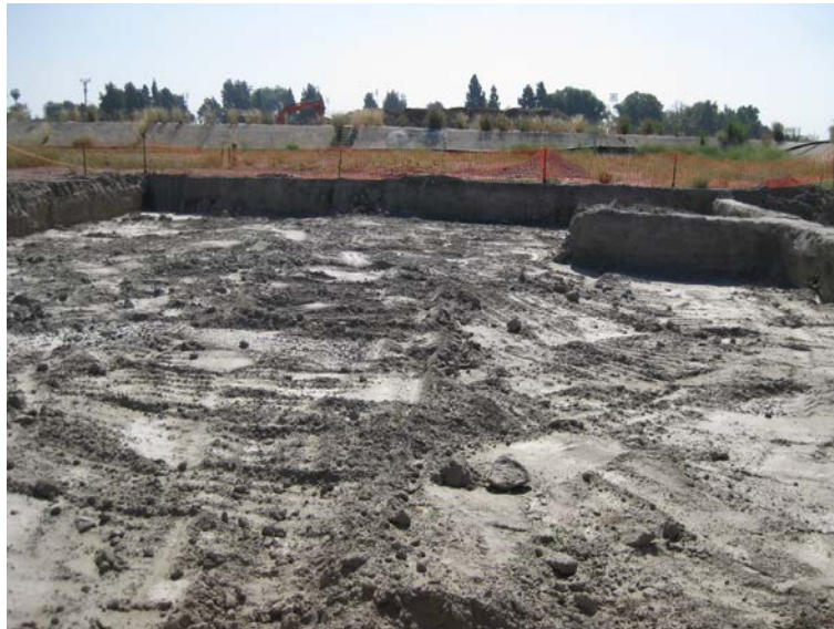
Photo 6: Excavation #8 prior to backfilling. View to the east.
