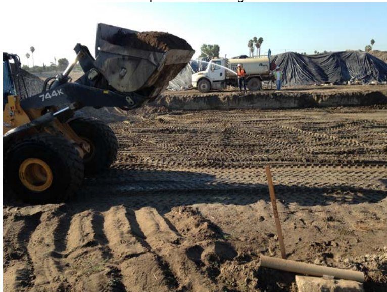
Photo 4: Excavation #2 during backfilling. View to the south.
