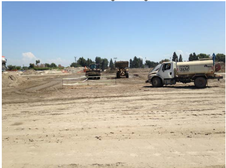
Photo 5: Excavation #2 post backfilling. View to the east.
