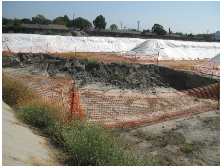
Photo 1: Excavation #1 prior to backfilling. View to the northeast.
