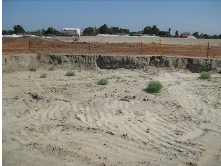
Photo 3: Excavation #2 prior to backfilling. View to the northwest.
